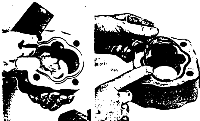
Fig. 14 Installing pre-greased "O" ring
